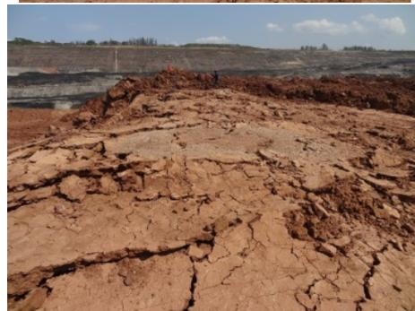
Figure 4 Blast#2 : Pile after blasting showing good fragmentation
