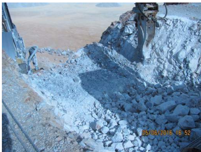
Picture # 5 - Road cut of depth 1,4 m
