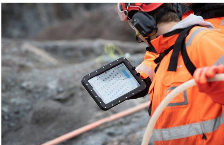
Figure 2. Use of ForAware's tablet during the explosive loading process.
