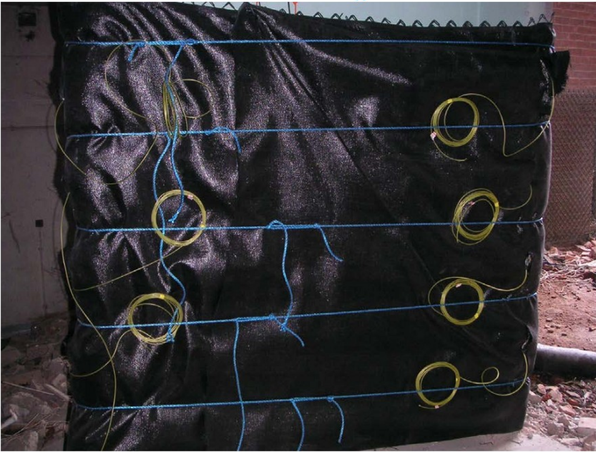
Column protection wrapping
