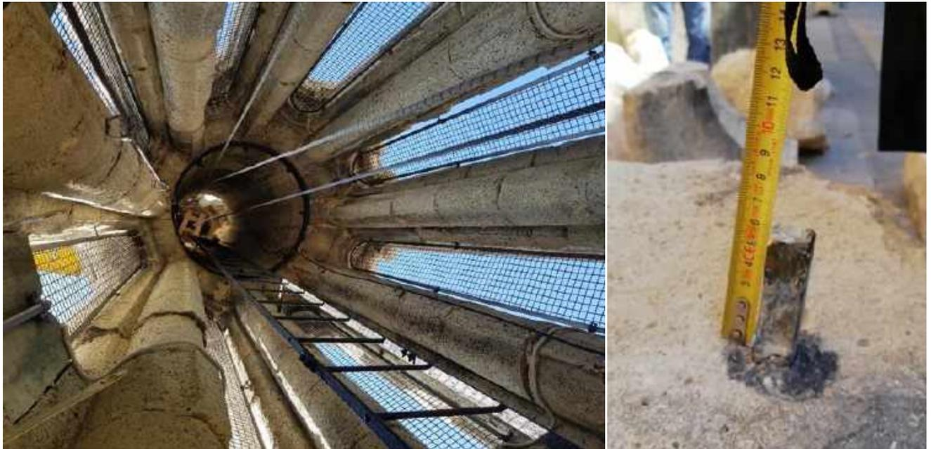
Figure 10. Steel wire rope and metal wedge.
