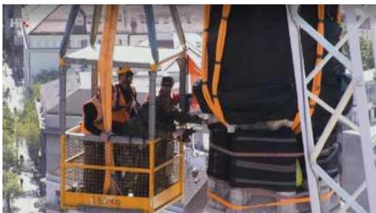
Figure 17. Preparation for blasting
