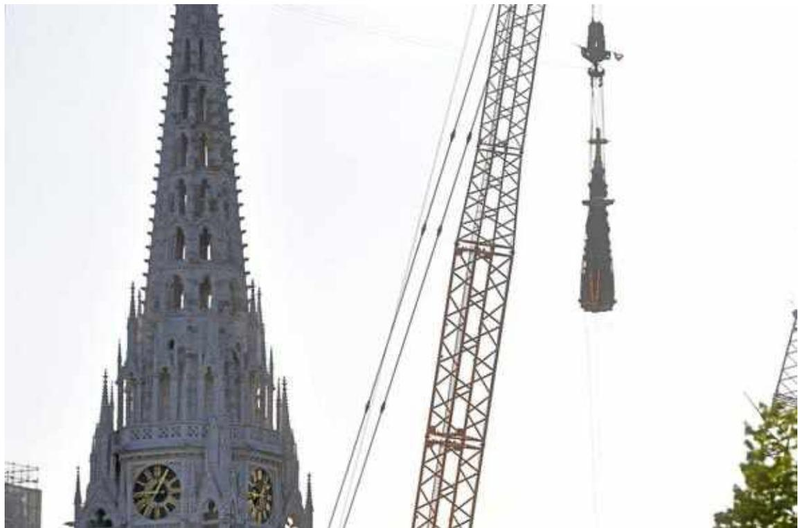
Figure 18. Blasting and lowering of northern tower (Photo: MORH/F. Klen)
