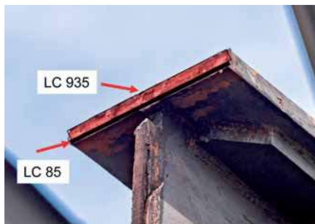
Fig. 11: Main wall after blasting - cutting surfaces upper chord
