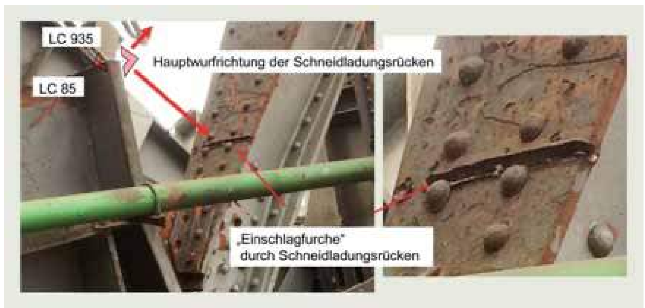
Fig. 12: Scattered flight of the copper pieces from the cutting charge
