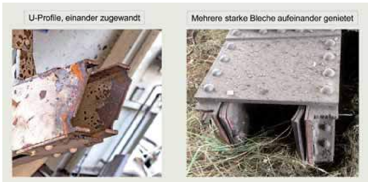
Fig. 8: Examples of cut profiles
