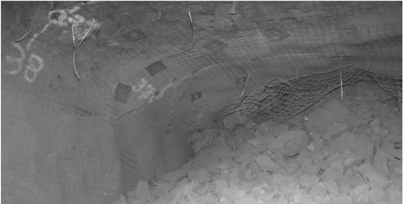
Figure 7. Multiple wireless charged rings are ready to fire as soon as needed, note strapping indicators
