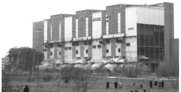
Figure 19. Water blasting boiler stanchions Thierbach.
