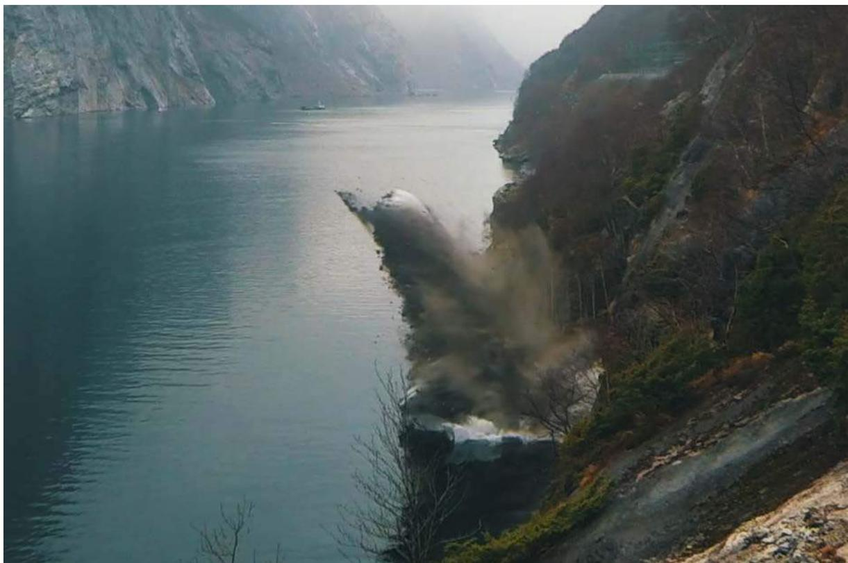
*Figure 9: No doubt that the blast in the outlet tunnel broke out into Lysefjorden (Lyse TV, 2017)*
