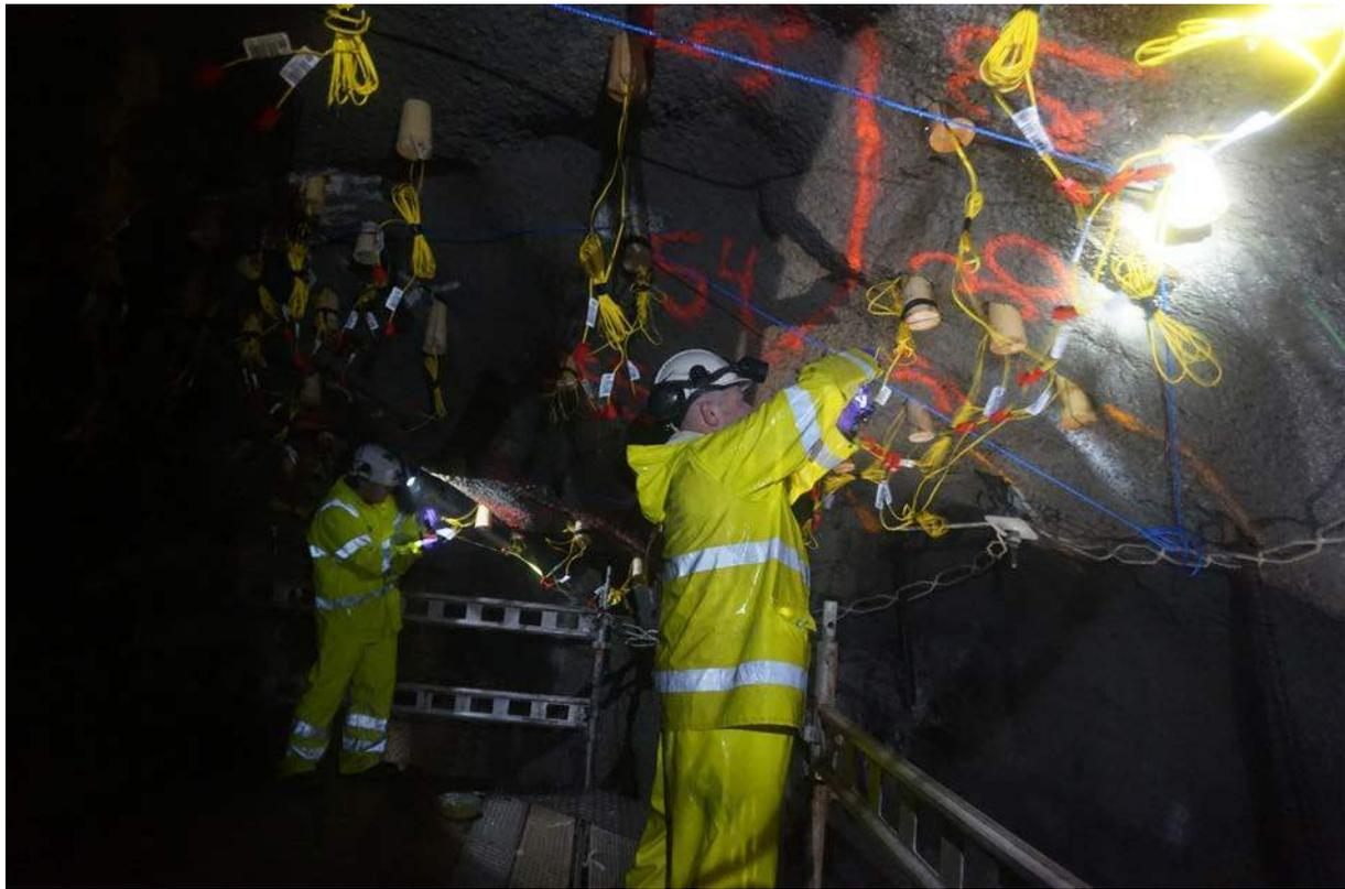
*Figure 8. Detonators are connected to bus wire and secured to the wooden plugs that locks the blast holes. Photo: Espen Hugaas*
