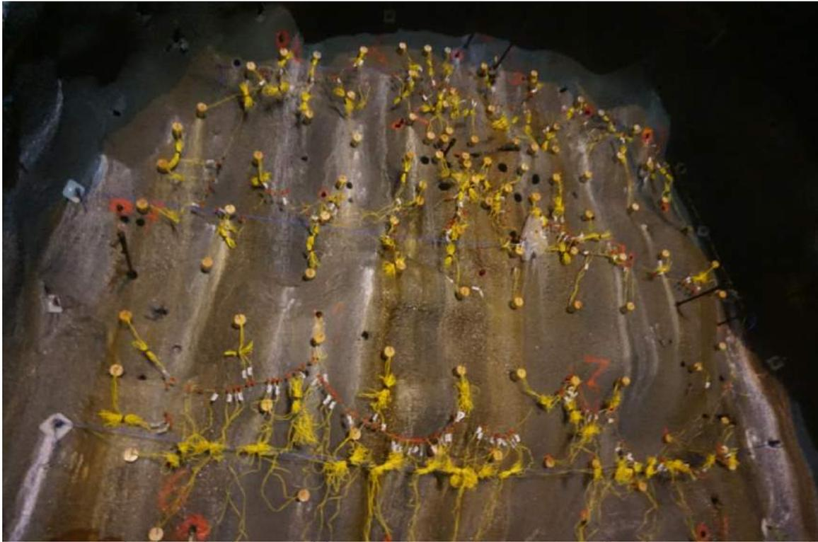
Figure 4. The breakthrough blast at the outlet into Lysefjorden charged and hooked up. Photo: Espen Hugaas
