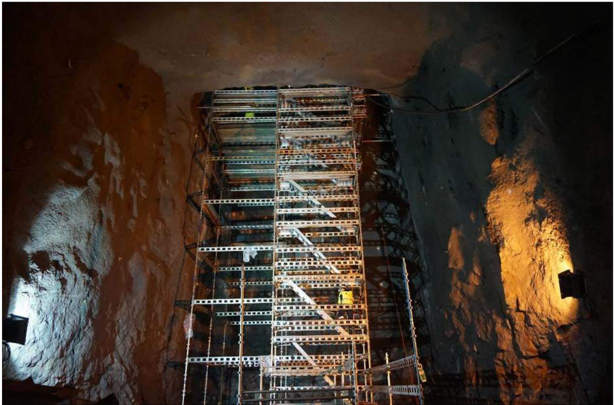
*Figure 6. Scaffolding installed under the lake Lyngsvatn break through blast.
