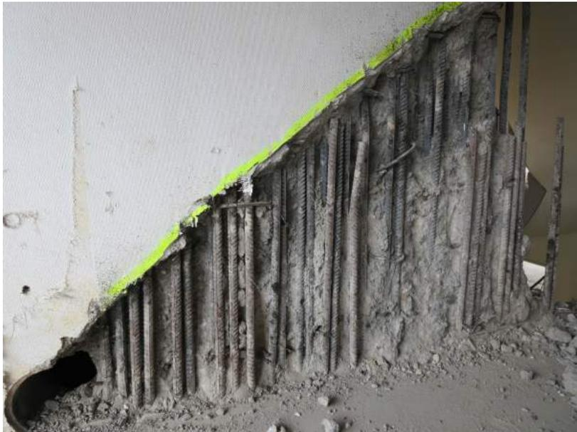
Fig. 6: Reinforcement in an falling slit to be chipped
