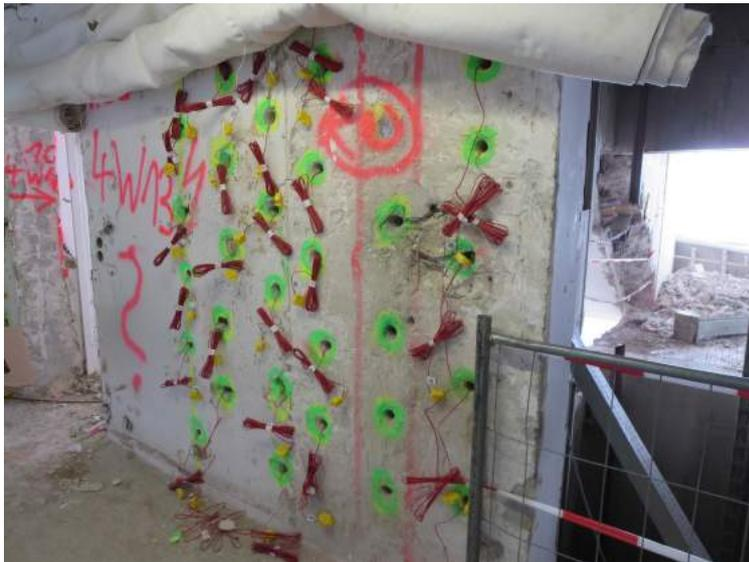
*Fig. 10:* Blasting unit on the fourth floor with electronic E-Star detonators
