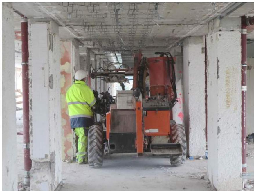
Fig. 3: Spot drilling the pillars using a Commando drilling unit
