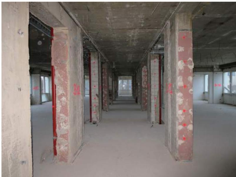
Fig. 2: Pillars laid open after gutting
