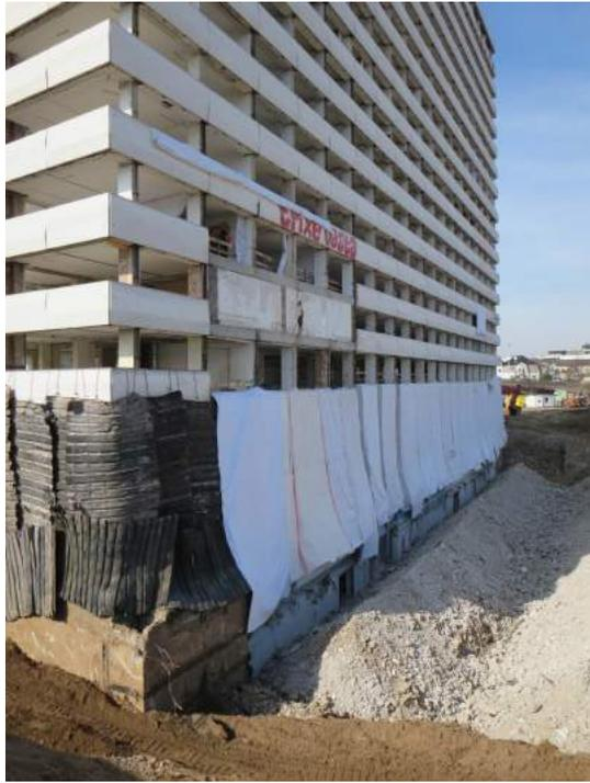
*Fig. 7: Sandwich covering and heavy blasting mats*
