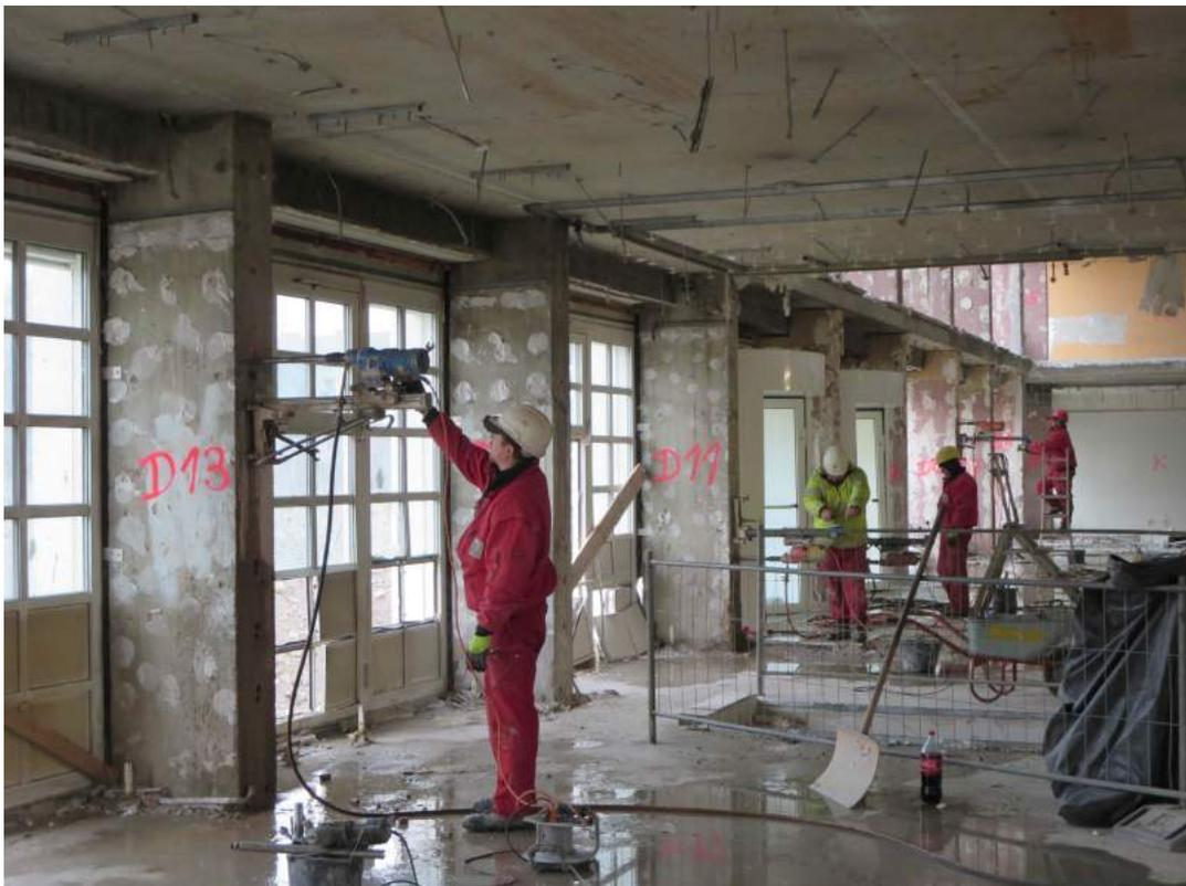
*Fig. 5:* Simultaneously applying multiple coring machines
