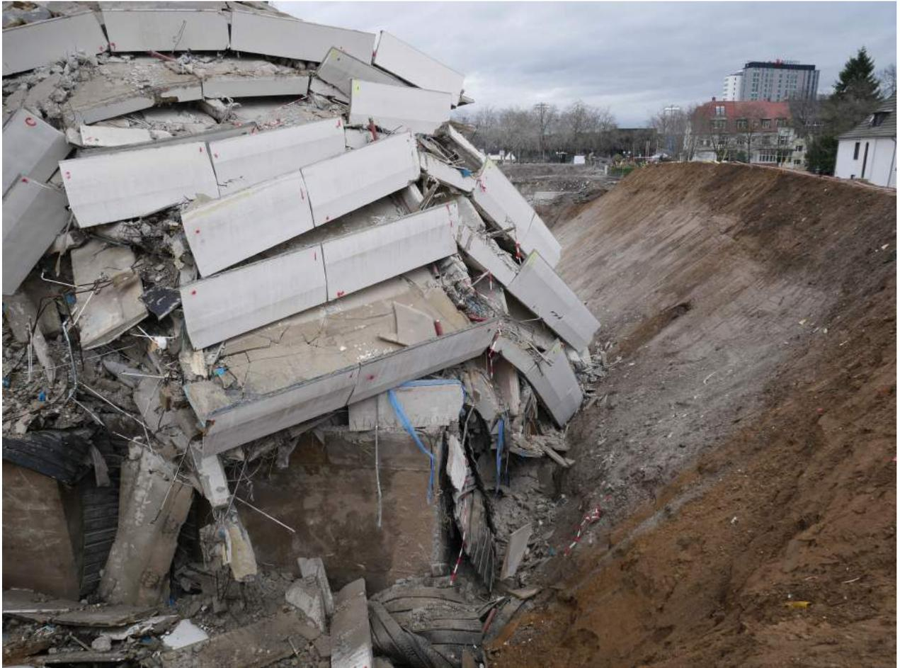
Fig. 12: Detailed view of the blasting result
