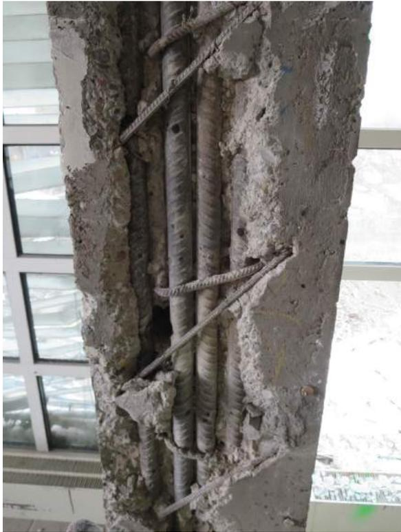
*Fig. 4:* Example of a pillar's rising reinforcement on the ground floor
