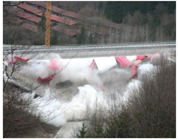
*Fig. 10b - 10c. Blasting the northern bridge*
