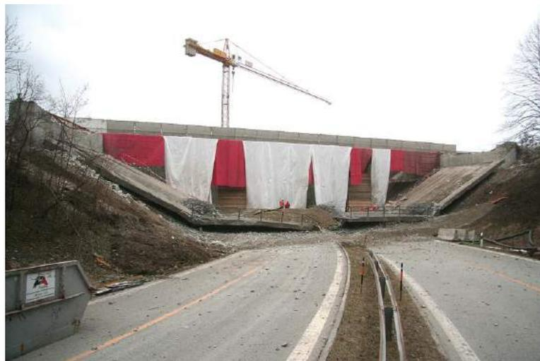
*Fig. 11. Northern bridge, blast results*
