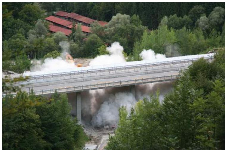
Following the necessary preparations, protection measures and charging, the southern bridge was blasted on 9<sup>th</sup> August 2012 (fig. 8a - 8c).
