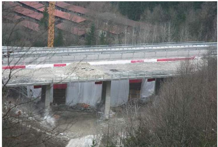
*Fig. 10a. Blasting the northern bridge*
