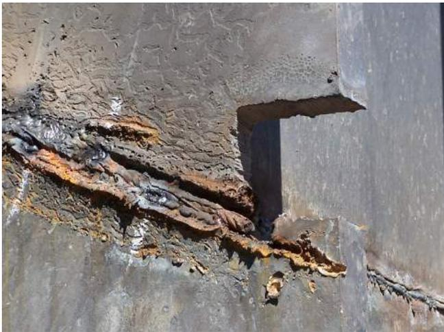
Fig. 7: insufficient cut after blast (attempt)
