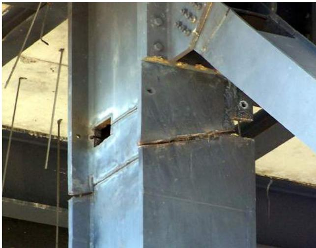
Fig. 5: improper cut
