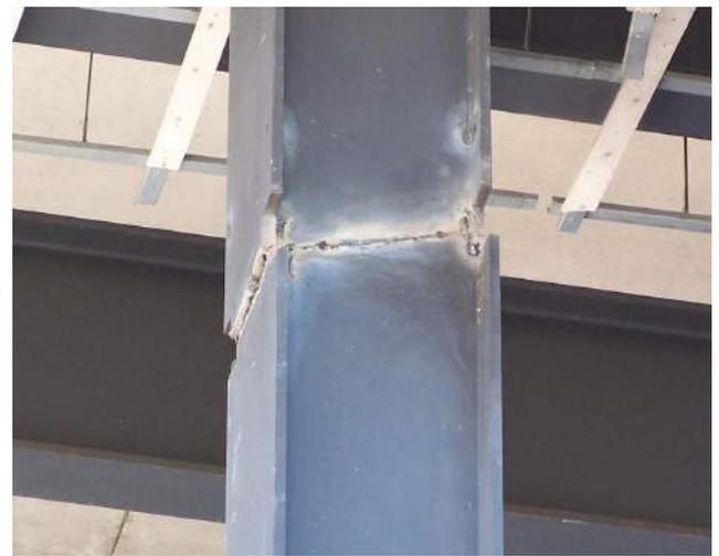
Fig. 6: improper cut
