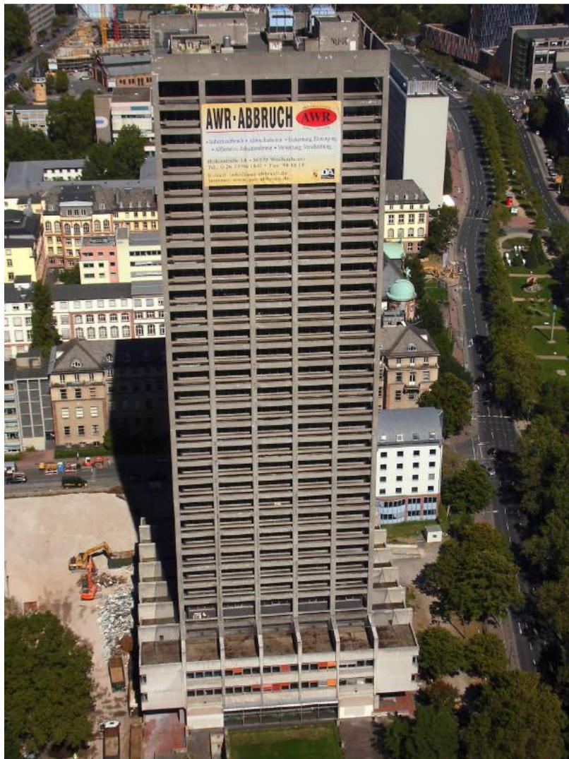
The basic principle of the blast demolition was a first vertical collapse of the skeleton part and a following folding of the core. The first vertical collapse was caused by blasting all columns in five floors. The three seconds later core folding completed the building drop down to an only 8 m high debris heap with a total length of about 100 m and a breadth of about 50 m.
